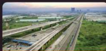
3 Exit Toll (KM 29, KM 31 & KM 34,7)
