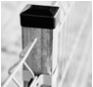
Anti Climb Perimeter Fencing
