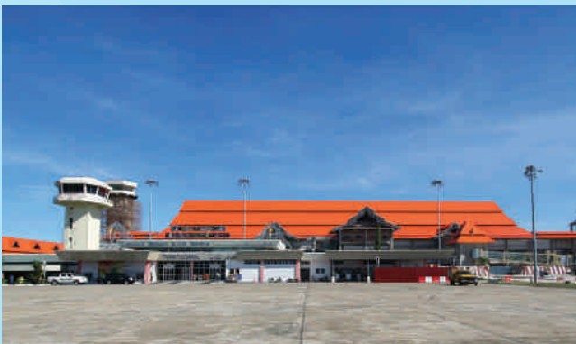
7 KM to Sultan Mahmud Airport
